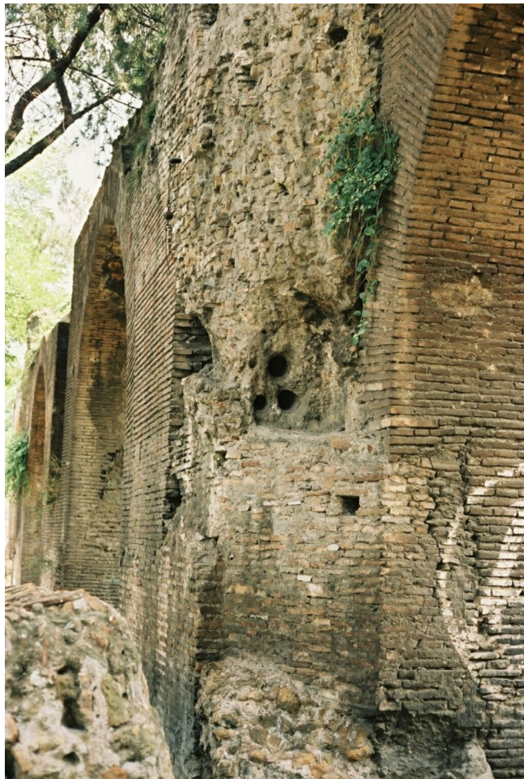
Figure D.20: Clay pipes in the Claudia ( http://www.romanaqueducts.info )
