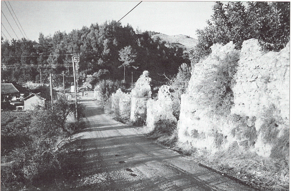
Figure 17 Mortared rubble wall, piers of low venter bridge.
