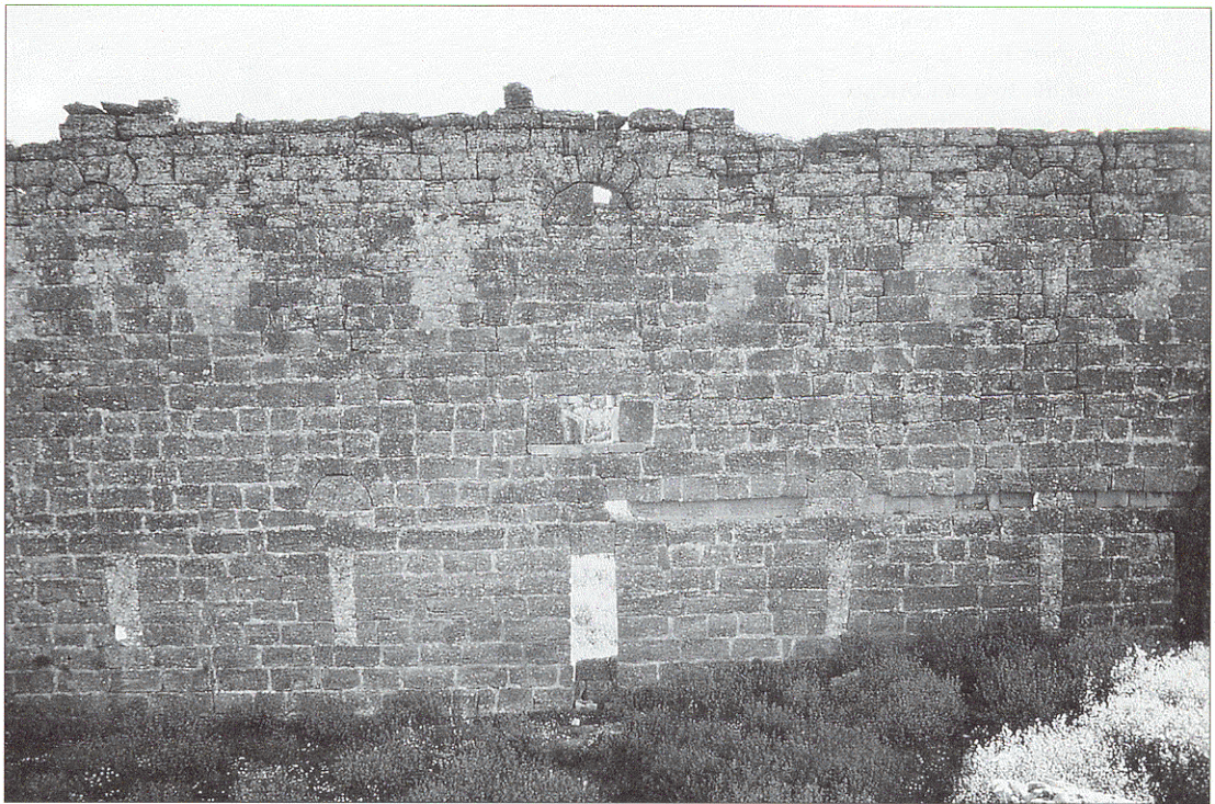
Figure 14 Backside of nymphaeum. Horizontal recess 5 m above ground level running from west side towards central niche.
