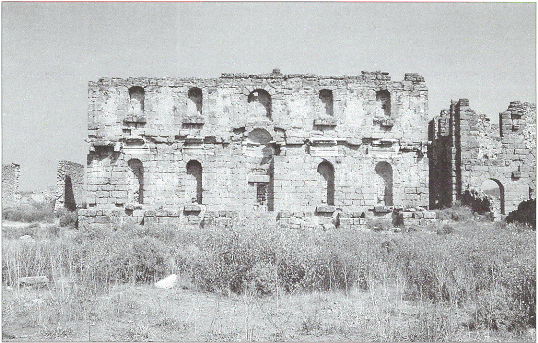
Figure 2 Façade of the nymphaeum on the acropolis of Aspendos. To the right: entrance hall of the basilica.
