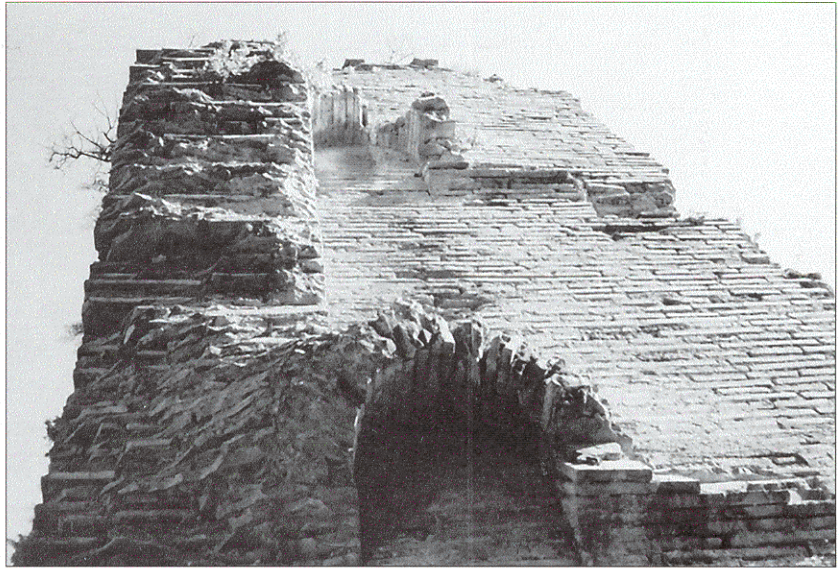
Figure 7 Inside wall of south tower adjoining south ramp.
