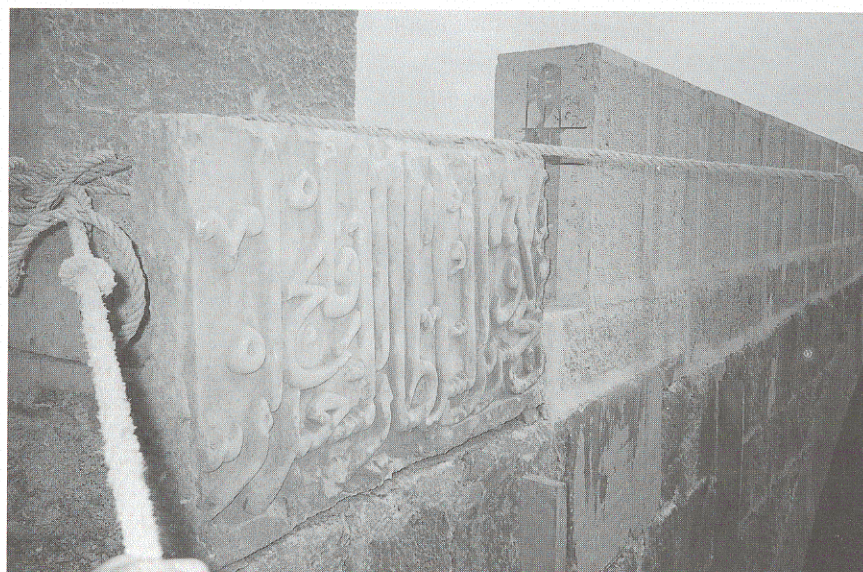
Figure 22 The Construction of new parapet with the Seljuk inscription (H. Franssen).
