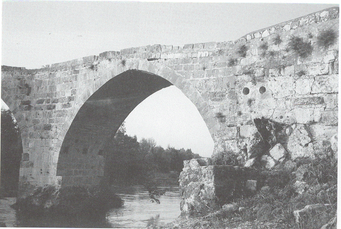
Figure 9-10 Pipe elements of the Aspendos siphon incorporated into the Seljuk bridge.
