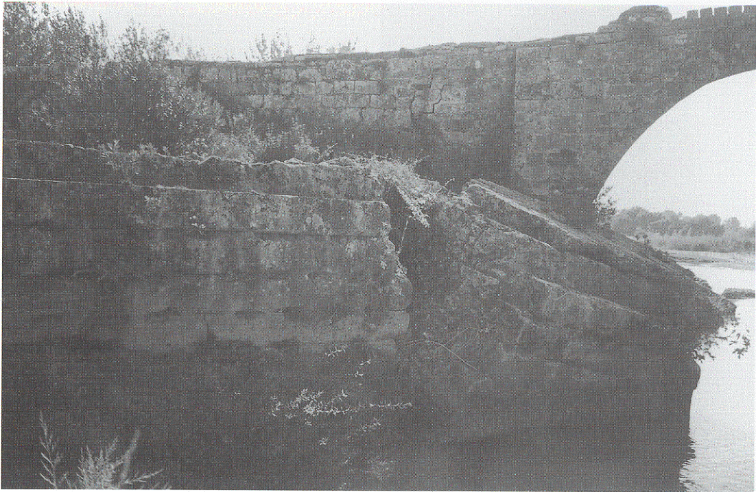
Figure 17 Remnants of the upstream mole of the Roman bridge, on the left side of river.
