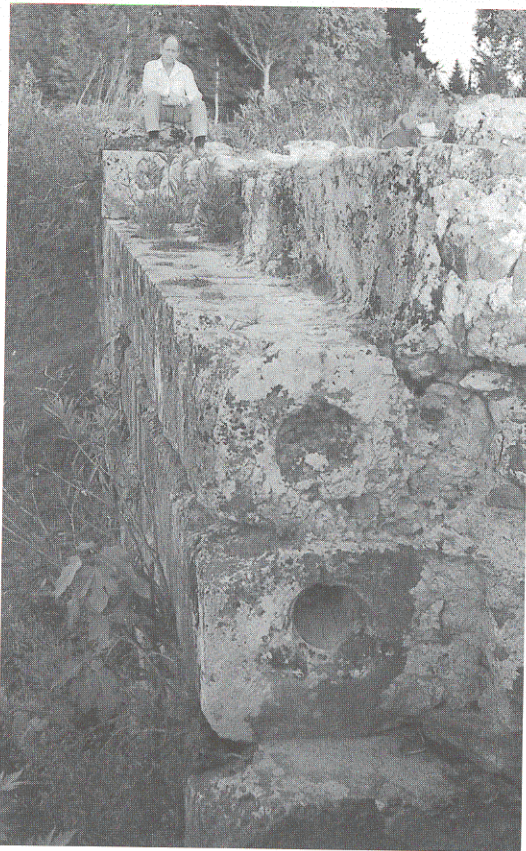
Figure 11 Pipe elements of the Aspendos siphon incorporated in the Roman mole.
