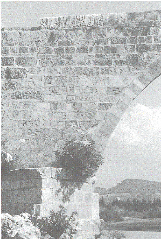
Figure 19 The Parapet with the Seljuk
