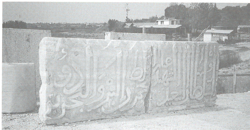
Figure 21 Two stone slabs with the inscription to be replaced in the parapet (H. Franssen).
