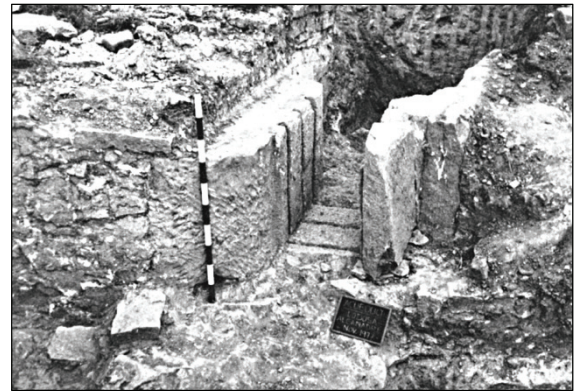
Calahorra (Spain): an aqueduct branch was equipped with three sets of grooves, probably a combination of two sluice gates and a filter screen (Casado 1983, pag. 516).
