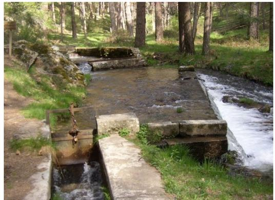
**Fig. 5: The start of the aqueduct of Segovia (Spain) should have been a river tap. At right a weir in the river Acebeda, in the front a sluice gate to direct the water via the aqueduct channel to the ancient city of Segovia (photo: Schram).**
