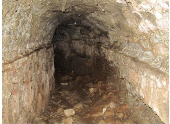
**Fig. 7: Inside the aqueduct channel. The floor and walls were covered with watertight plaster. On the ceiling one can see the imprints of the formwork used during the construction. (Aqua Anio Novus, S of the Ponte degli Arcinelli, S of Tivoli, Italy). (photo: Schram).**
