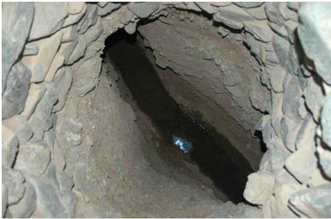
**Fig. 2 (top):** View into the channel of a qanat, seen from the top of a vertical access shaft (source: Wikipedia).
