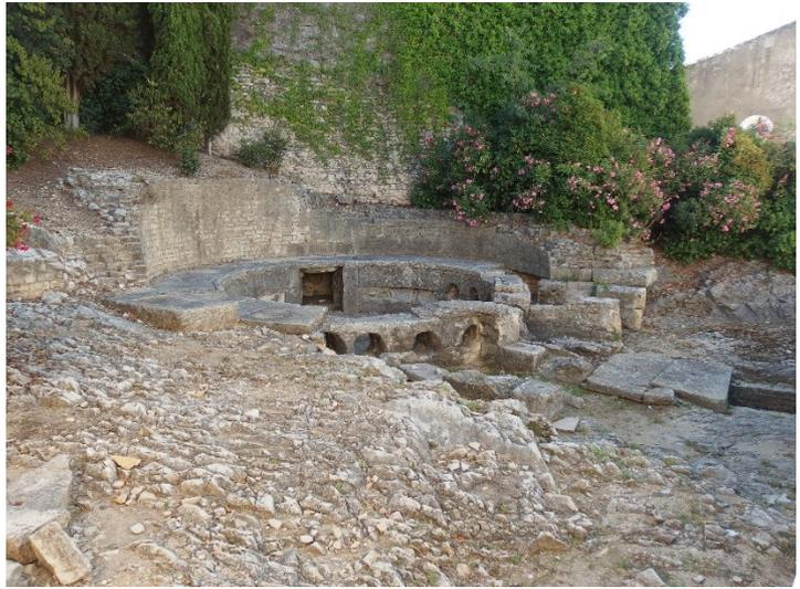
**Fig. 10: The well-known water distribution basin (*castellum divisorium*) of the aqueduct of Nîmes (France). The inlet in the background may have been equipped with a kind of sluice gate. In the front some of the in total 10 openings for (ceramic ?) pipes to distribute water to the users (Photo: Hauke Krebs).**
